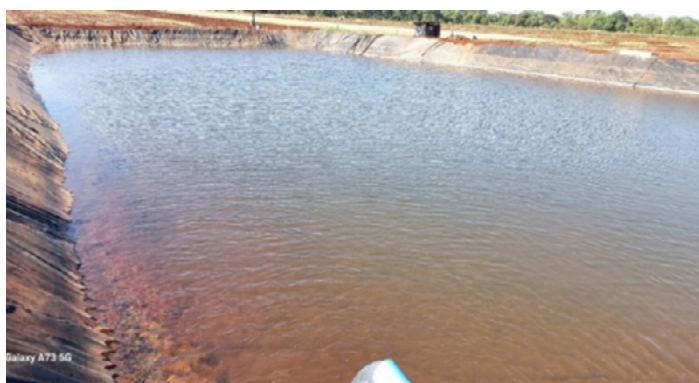
Figure 12. A 2 000 m3 reservoir constructed at the station
