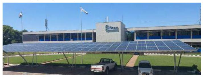
Fig 2.5.2 The spectacular Kutsaga solar 78 solar panel carport – 48KW system powering the two Administration block floors
